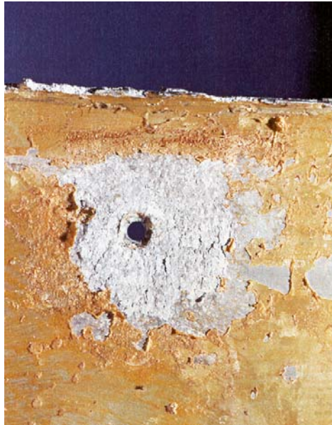
Crevice corrosion under a floor cover
